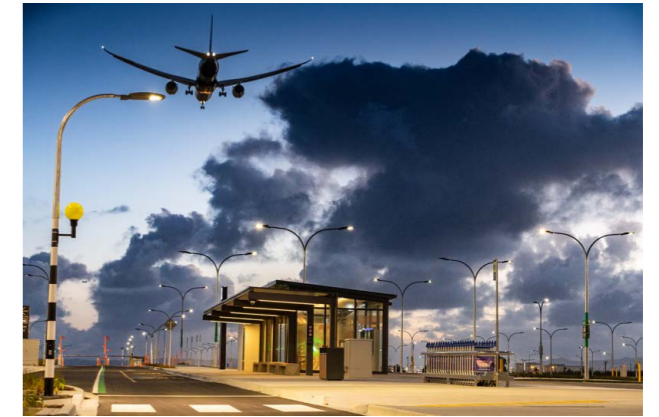
4 Park & Ride South opened on SH20B/Puhinui Road in early June 2024.
