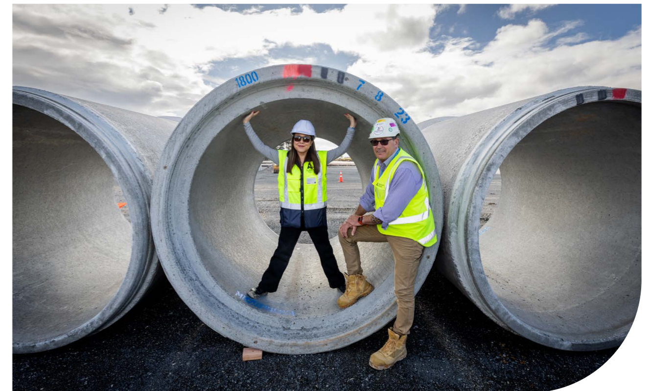
Pre-implementation Programme Manager Adrienne Khor and Mark Blanchard, Construction Operations Manager, demonstrate the size of stormwater pipes installed as part of a 3.5km network.
