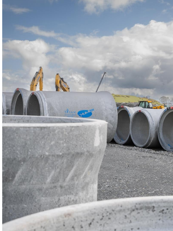
Stormwater pipes awaiting installation
