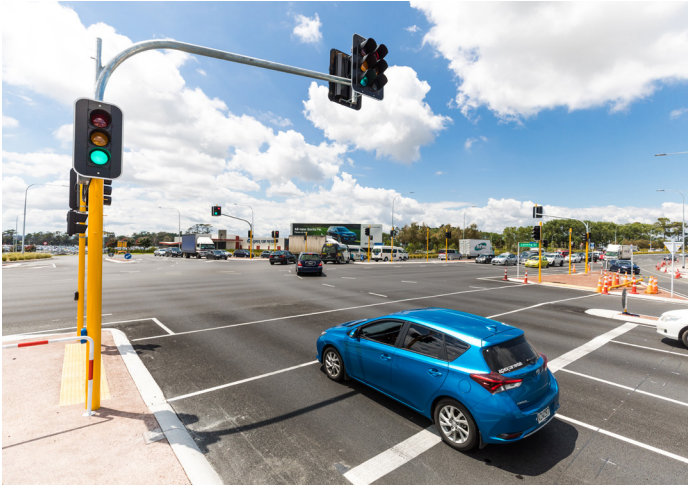
Completion of the signalisation of the Landing Road intersection.
