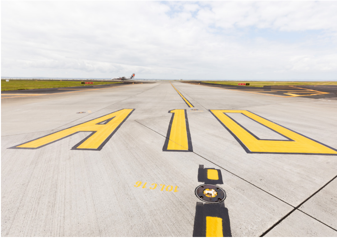
Airfield slab replacement work completed – 20,000 tonnes of concrete poured.
